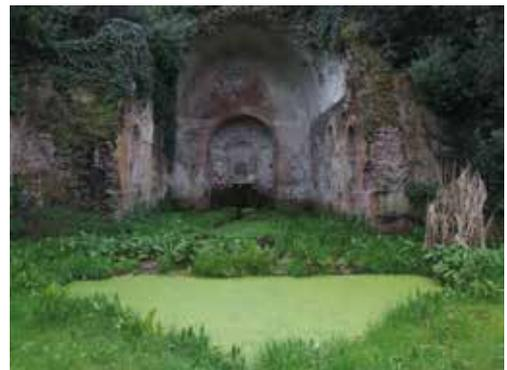
The architectural structure of the building can be easily recognized thanks to the restoration carried out in 1999. It consists of a big rectangular hall, with a niche at the bottom and three smaller niches on both lateral walls, everything built in "opus mixtum", with opus reticulatum and opus latericium. This building technique dates the building back to the half of the 2nd century AD.
