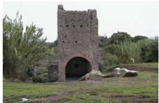
The construction, which over the centuries was restored several times, maintained a square plan with several storeys divided by wooden floors. Walls are lined with Peperino blocks, alternating in some areas with yellow tuff blocks.
